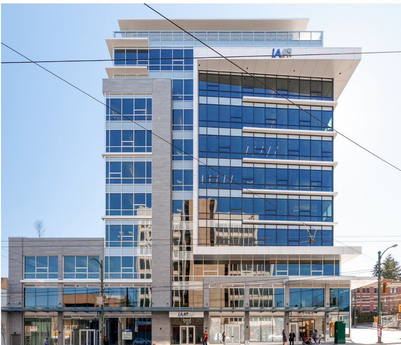
Above: The exterior of iA Financial's Vancouver Office, 988 West Broadway
